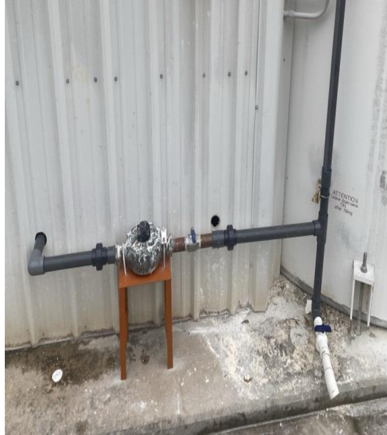
*Pictured above: is a lime spill due to fill valve getting cracked open; and new fill valve placement on outside of lime building.
