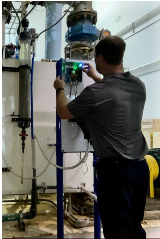
*Pictured above; Clay Stuart, installs new data recorders in Swan turbidimeters.
