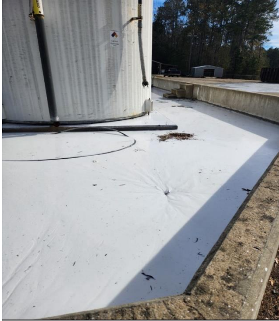
*Pictured above: is a lime spill due to fill valve getting cracked open; and new fill valve placement on outside of lime building.
